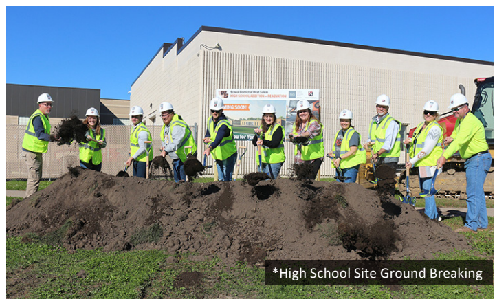
*High School Site Ground Breaking
